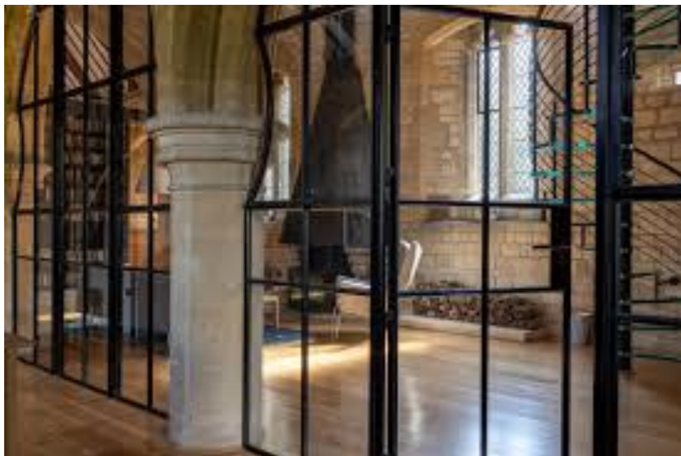
Similar sensitive glass insertions between columns to separate Aisle from Nave
