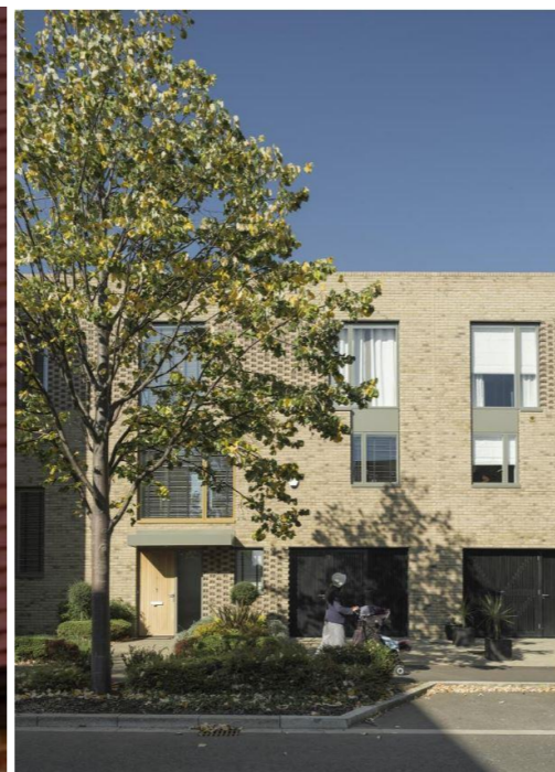
Front Elevation of a typical St. Kevin's townhouse terrace showing warm terracotta brick and protruded brick detail
