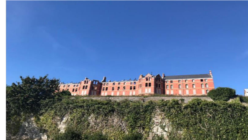
St Kevin's Hospital – RPS ref. no. PS1154 1
